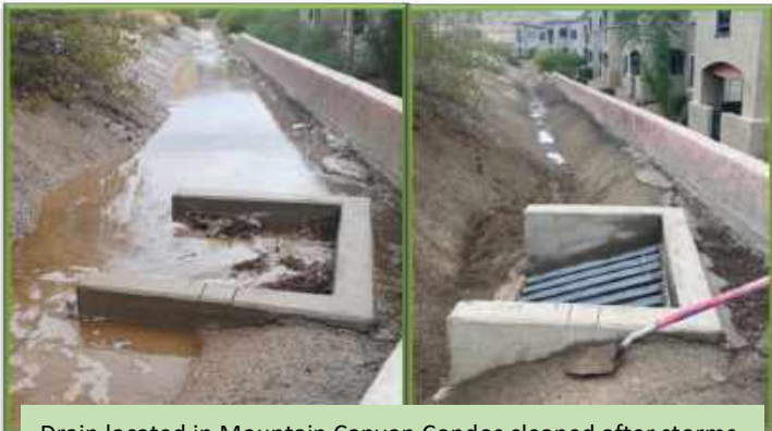
Drain located in Mountain Canyon Condos cleaned after storms
