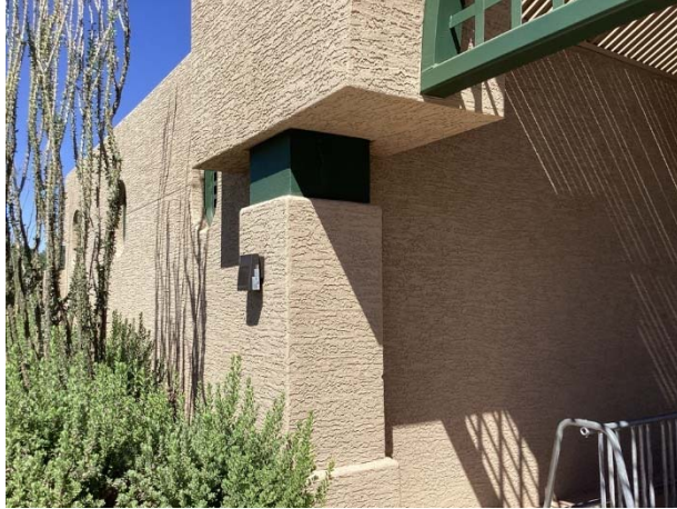
Stucco wall finishes at rec 3
