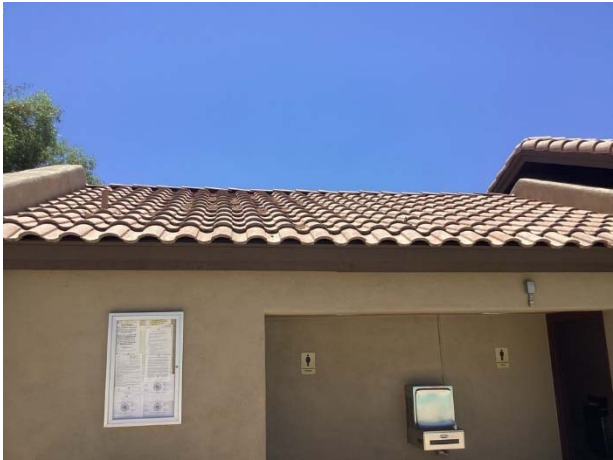
Concrete tile roof
