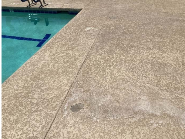
Textured coating delamination at rec 1
