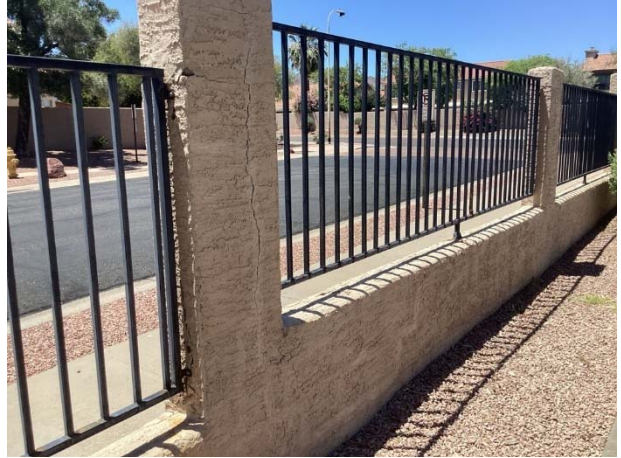
Wall stucco cracks
