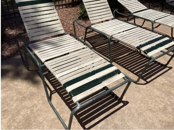
Frame finish deterioration
