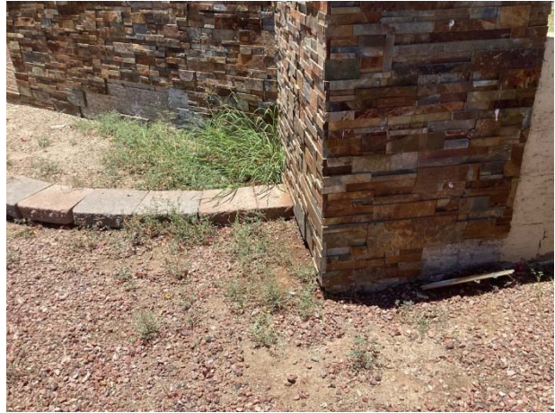
Delaminated stone tiles
