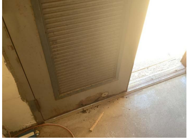
Rust at pool 3 equipment door
