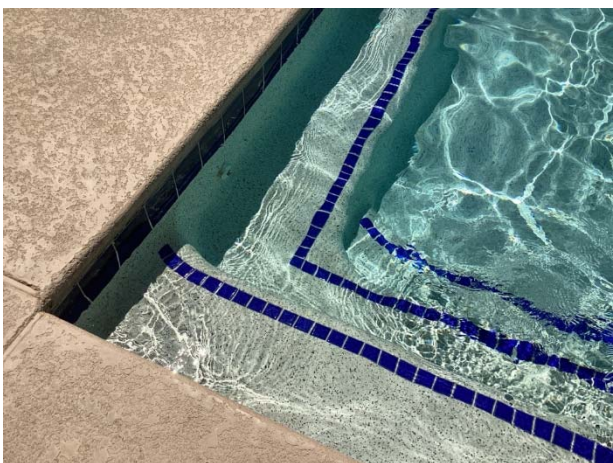
Pool plaster finish with tile perimeter at rec 2
