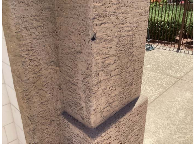
Stucco damage at rec 3
