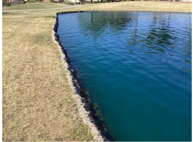
Concrete bulkhead/liner
