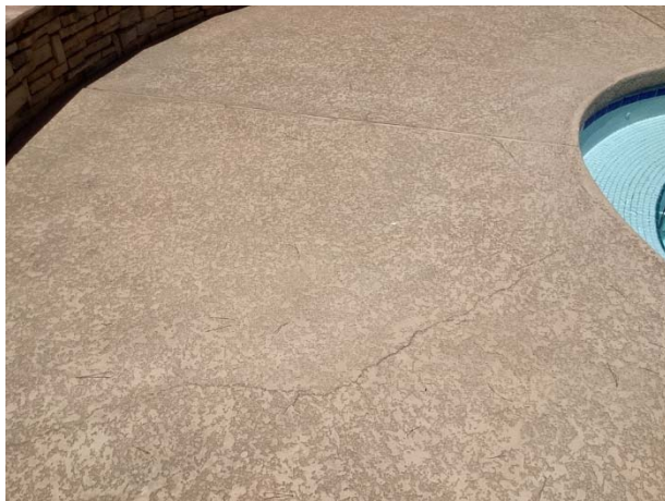
Coating cracks at rec 1
