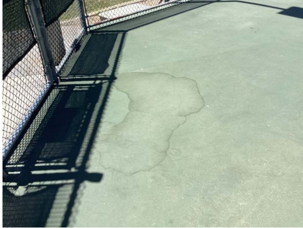
Prior ponded water evident near gate entry at rec 3
