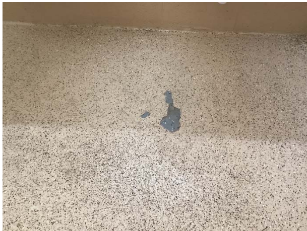
Epoxy flooring delamination
