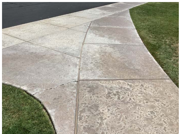
Concrete sidewalk with minor cracks at rec area
