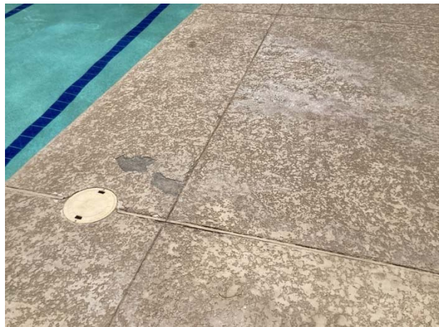
Textured coating delamination at rec 1
