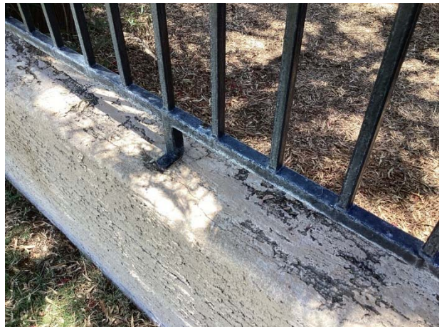
Paint finish deterioration
