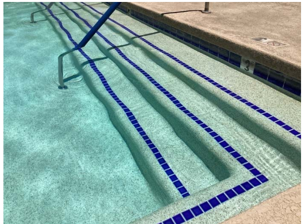
Pool plaster finish with tile perimeter at rec 1
