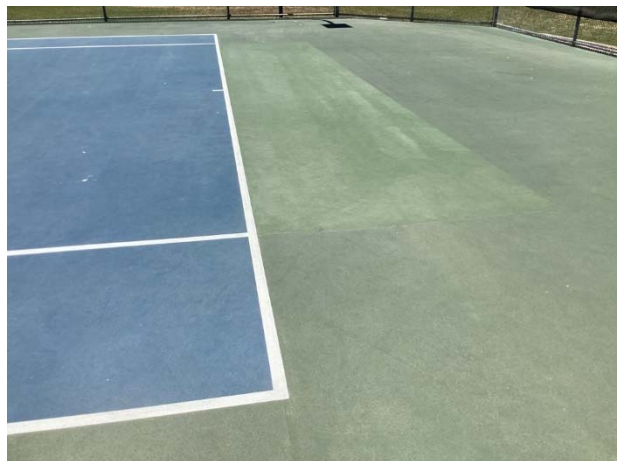
Previous repair or partial color coat at rec 3
