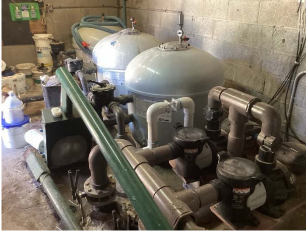
Pool pumps and filters at rec 1
