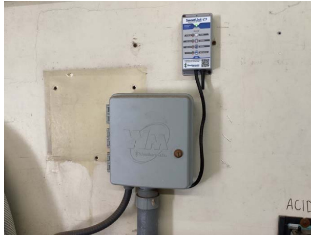
Irrigation system controller
