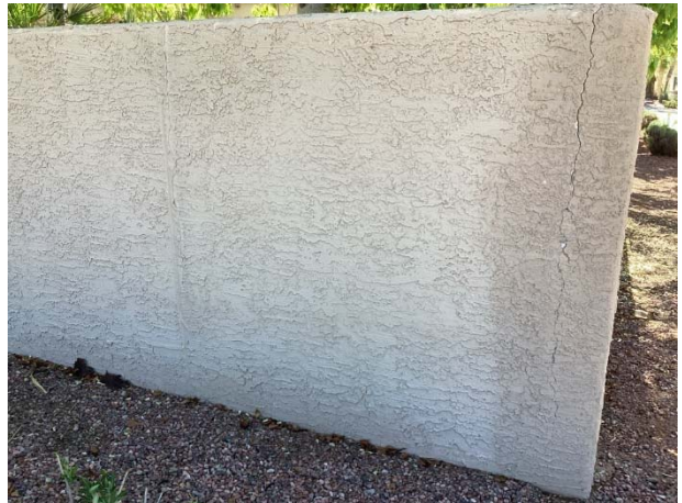
Wall stucco cracks
