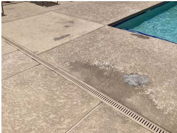
Textured coating delamination at rec 3
