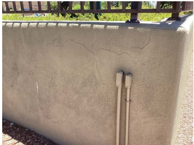
Stucco cracks at rec 1
