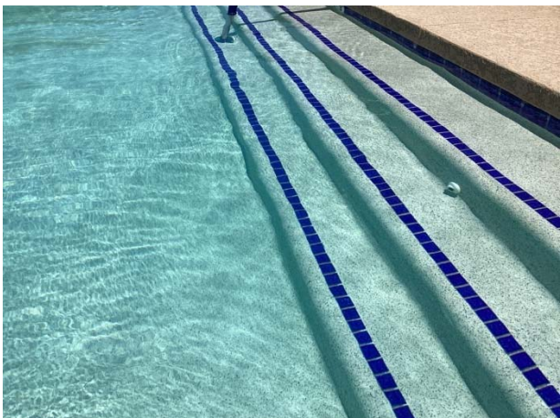
Pool plaster finish with tile perimeter at rec 3
