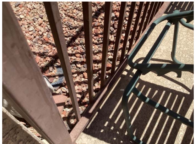
Fence finish deterioration at rec 2
