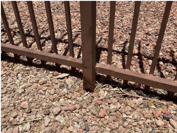
Post corrosion at rec 1
