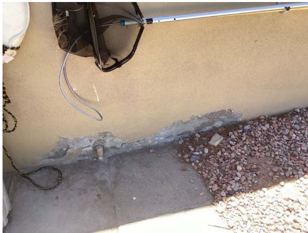
Stucco coating deterioration at rec 1
