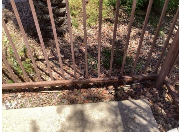
Fence rust and corrosion at rec 2
