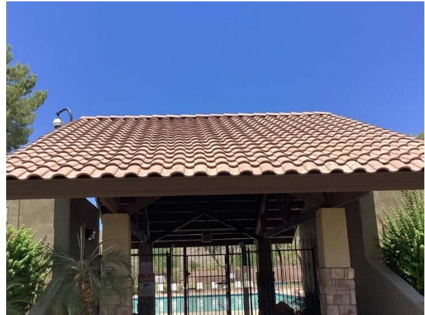
Concrete tile roof
