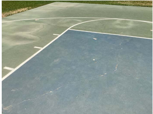
Concrete cracks and previous ponded water evident
