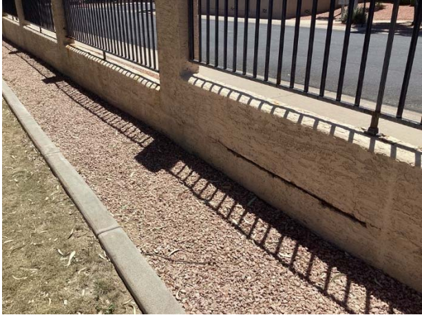
Wall stucco cracks and rust
