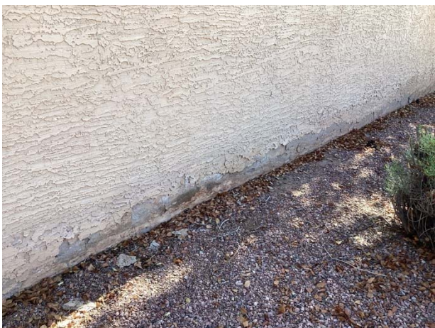
Wall paint finish deterioration along bottom
